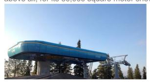
yet another attraction with the new CD8 Kungsliften. The new ropeway impresses with a higher transport capacity of up to 4,000 people an hour and the environmentally friendly, gearless LEITNER DirectDrive system. Kungsliften replaces three old ski lifts, two of which are being moved by LEITNER ropeways to another site in the ski resort.
