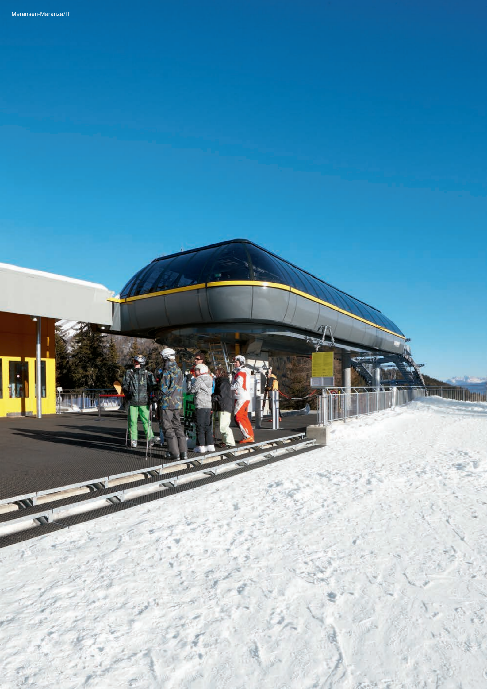
Karlesjochbahn, Feichten im Kaunertal/AT: - 8-passenger gondola lift with heated seats
