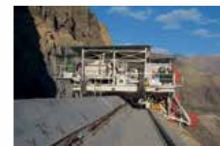
1997 Blondin barrage Karun III – Iran
